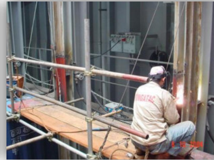
Cell Guide Repair
