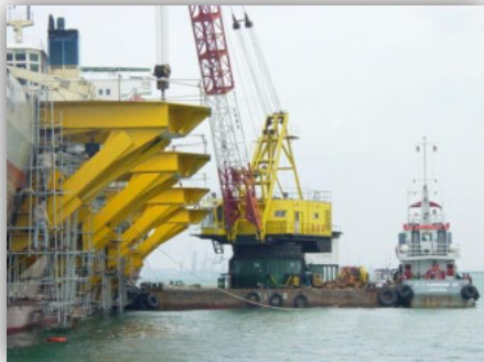
Installation of Outriggers
